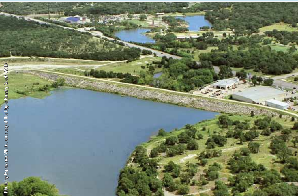
Upper Brushy Creek WCID's Dam No. 6 in Cedar Park.
